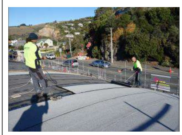
Installation of Duo cap sheet
