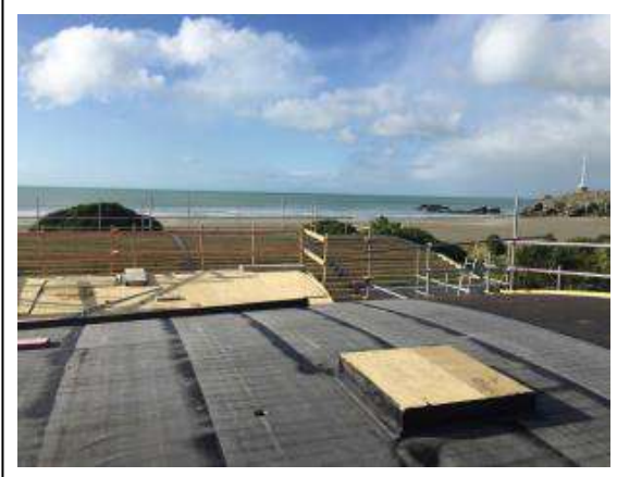
Installation of Duo base sheet over plywood
