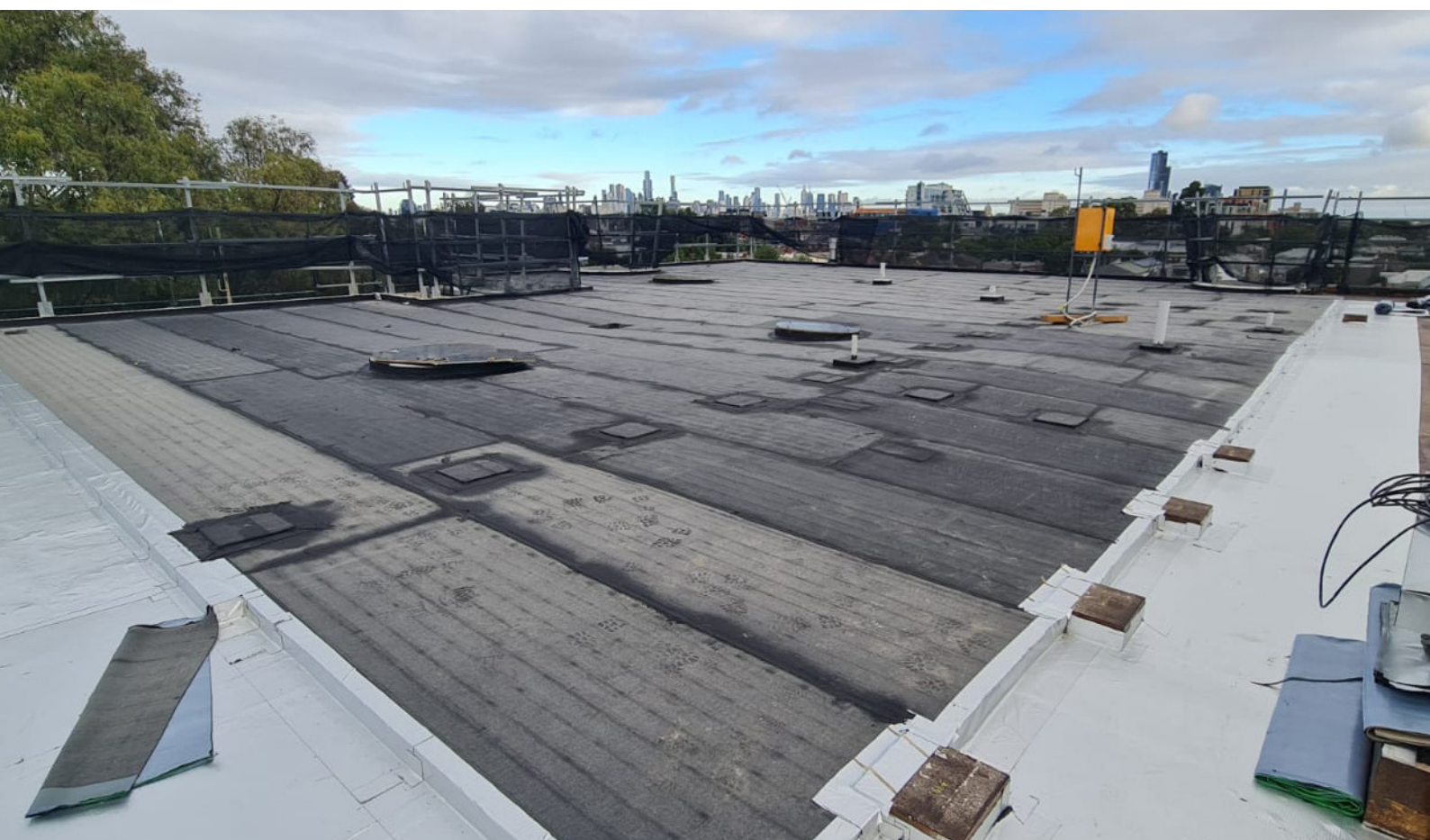
Base Sheet installation
