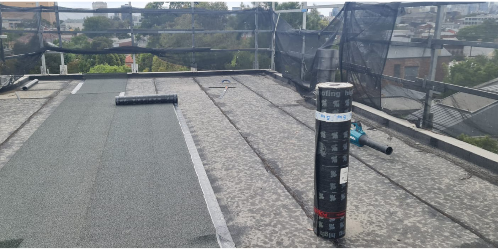
Cap Sheet installation
