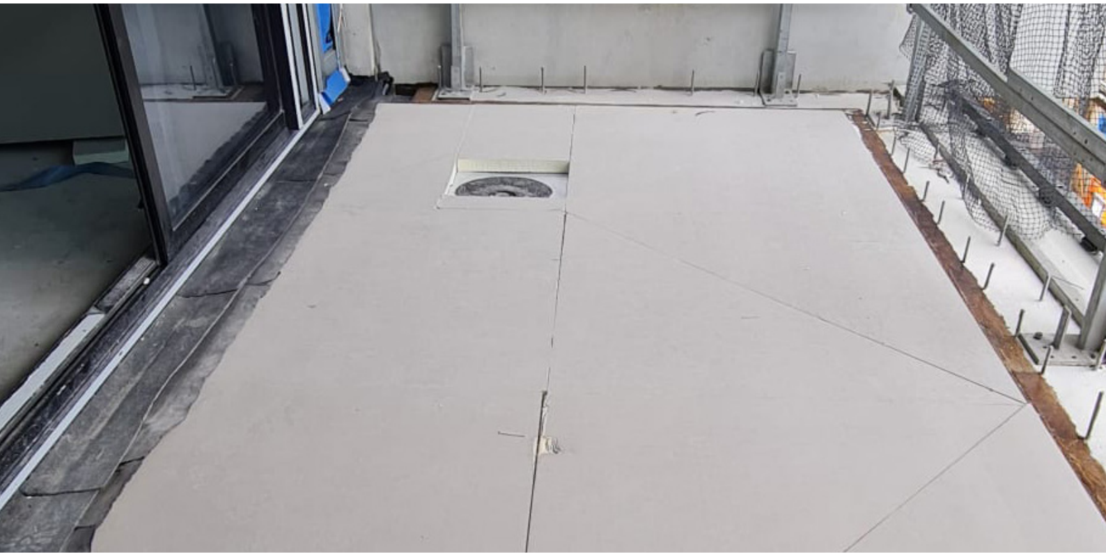
Insulation installed in Balcony
