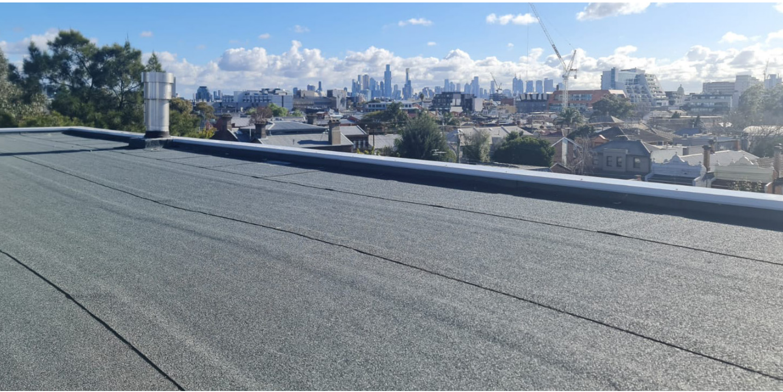
Cap Sheet installed
