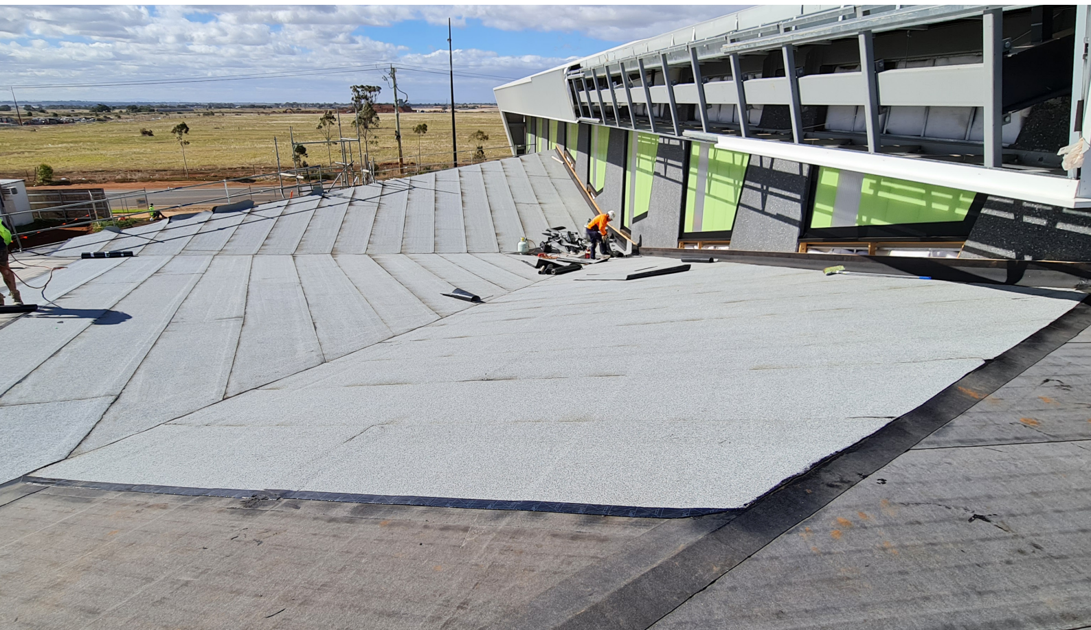
Cap Sheet installation
