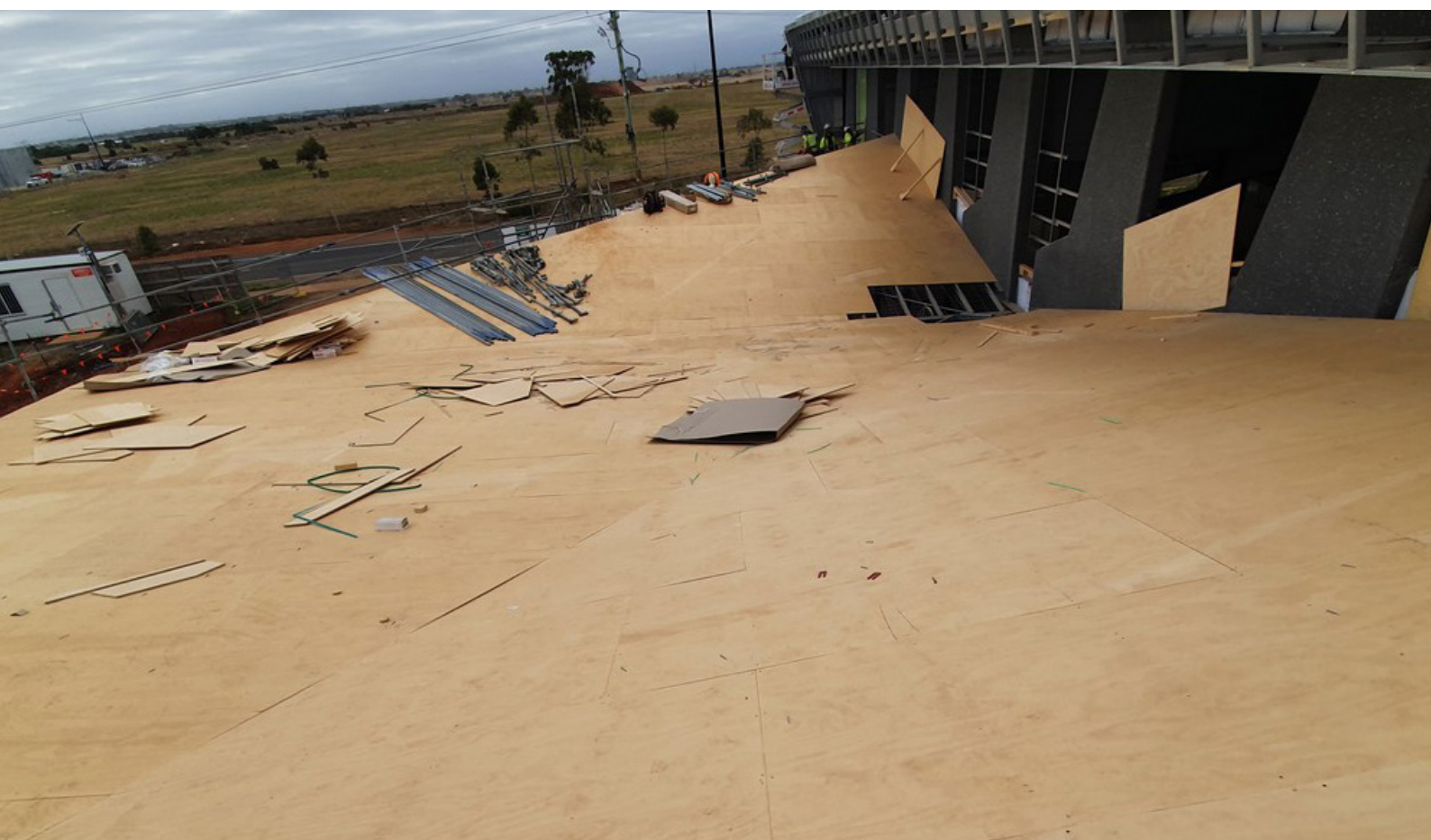
Preparation for insulation
