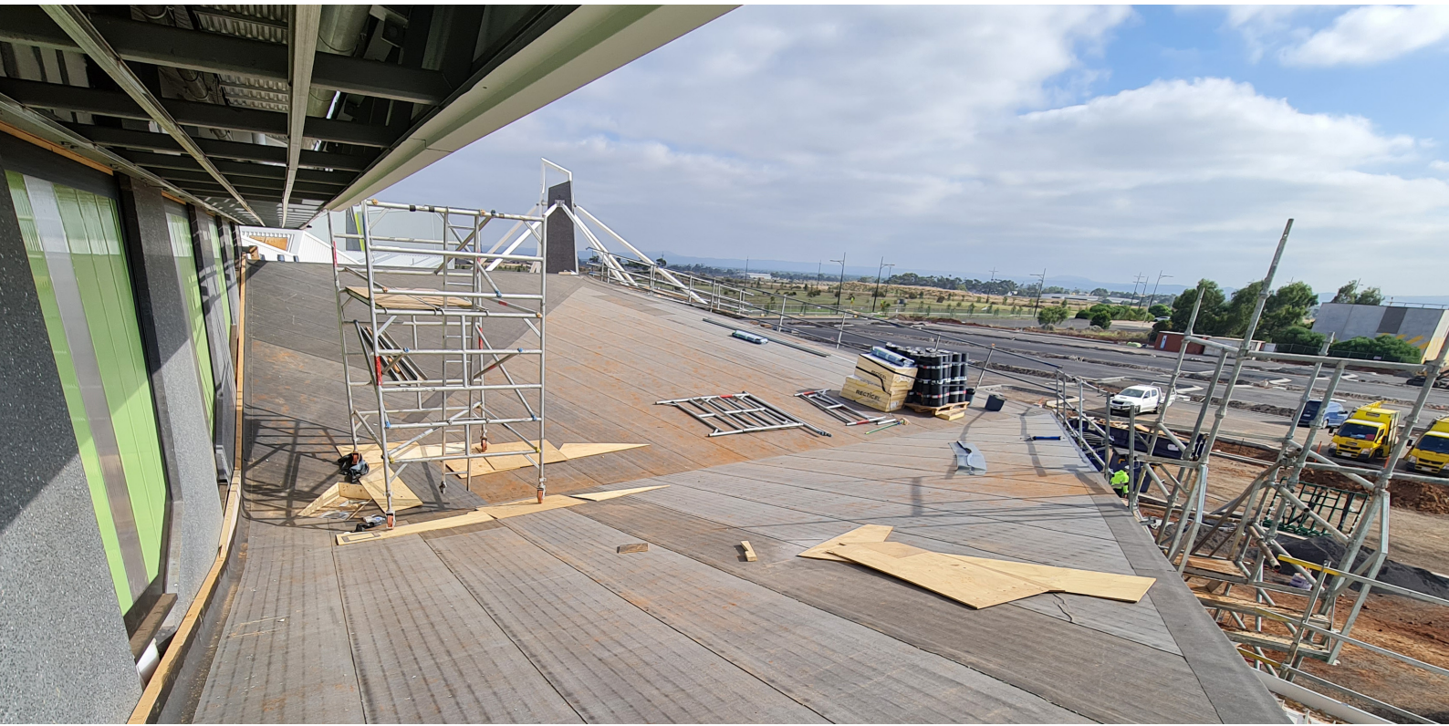
Base Sheet installation
