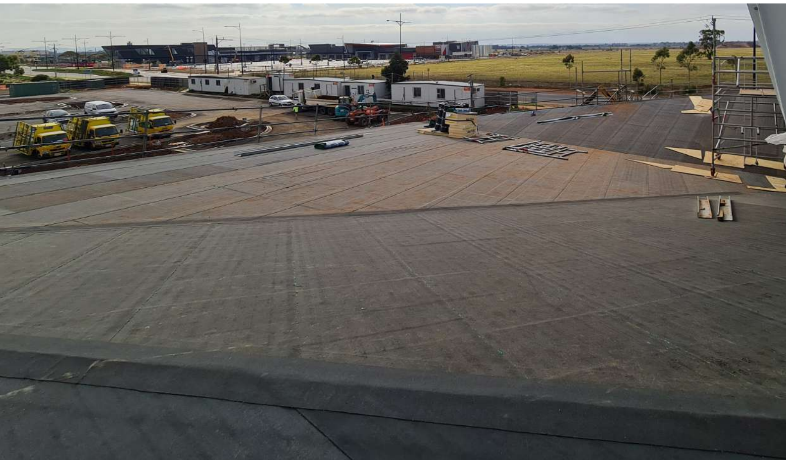
Membrane Installation
