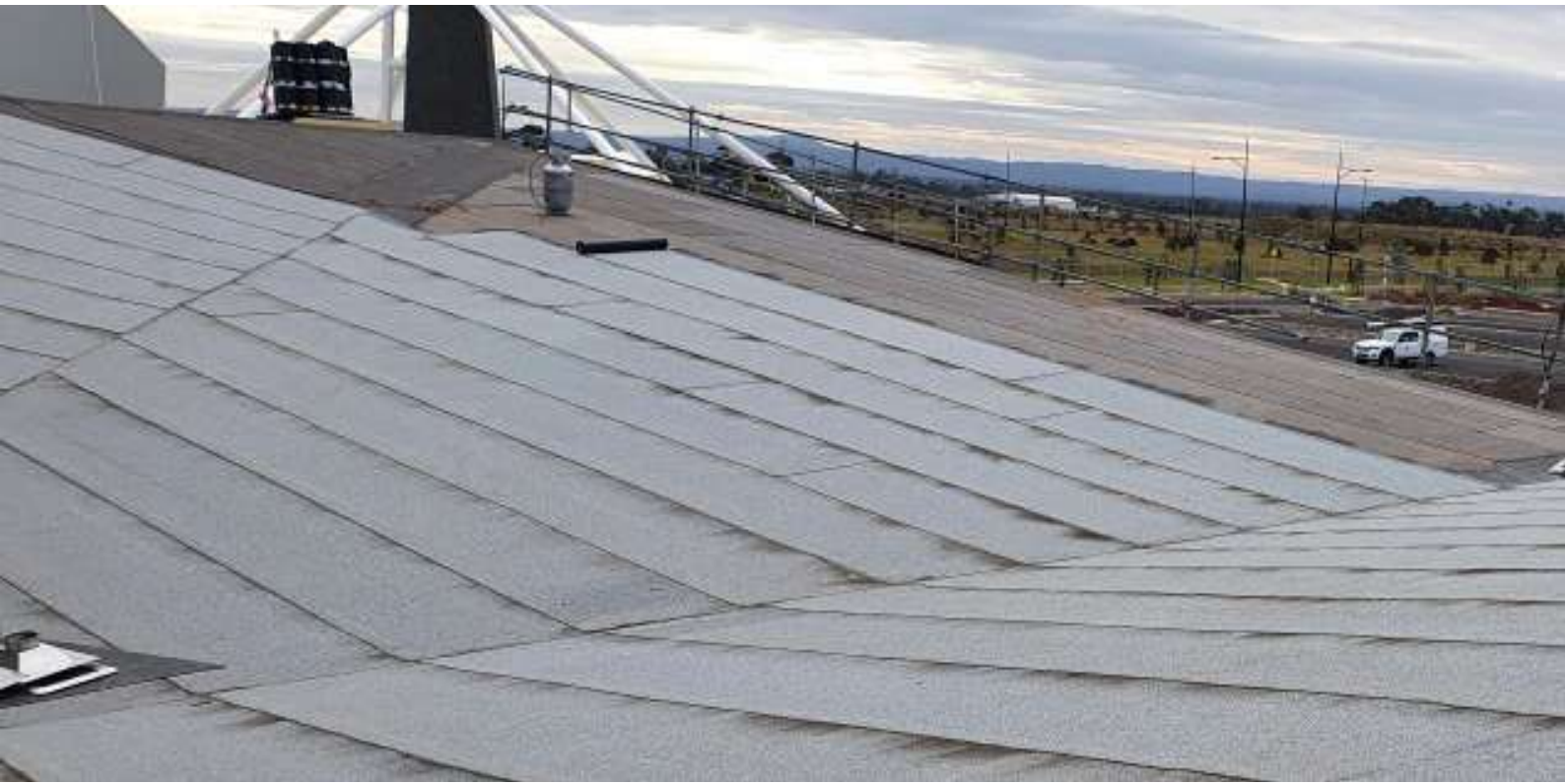
Membrane Installation
