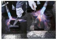
3- Weld the flange onto the 1st waterproofing layer.
